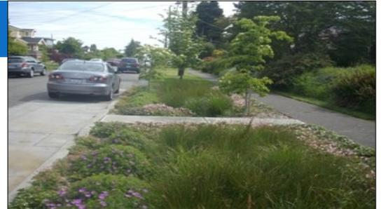
**This Ballard rain garden - a type of natural drainage - helps to keep stormwater out of the sewer system and prevent raw sewage overflows into Salmon Bay.**
